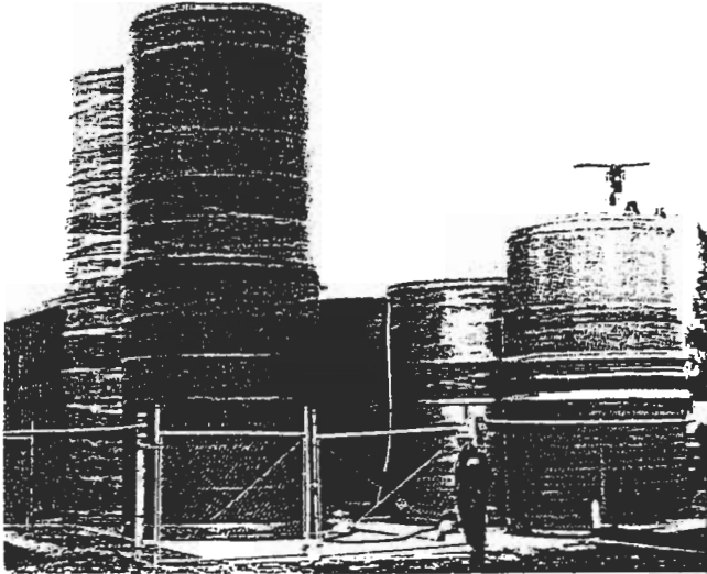
Liquid fertilizer storage facilities consist of large tanks of metal or plastic. The basic materials are usually mixed to the desired analysis just before application.
